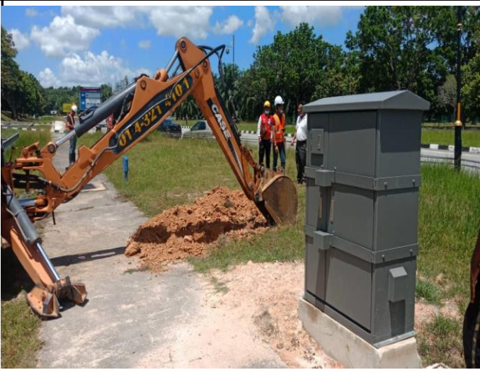
doing check underground cable
