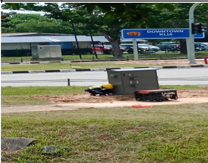
to supply and install controller and earthing controller
