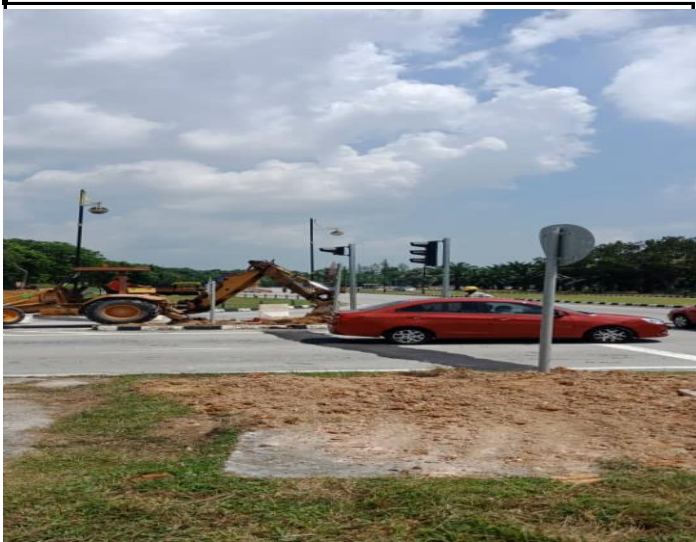
completed to install g.i pipe and pole and aspect
