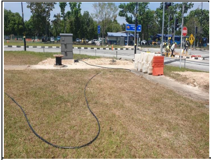
to supply and install cable amour cable
