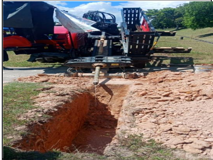
prepare lay the pipe
