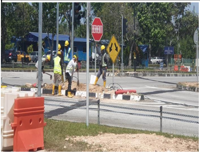
install cable pit, detector pit and completed to install g.i pipe
