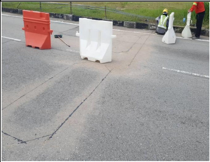
completed to lay the loop cable
