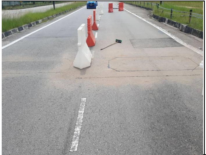
completed to lay the loop cable
