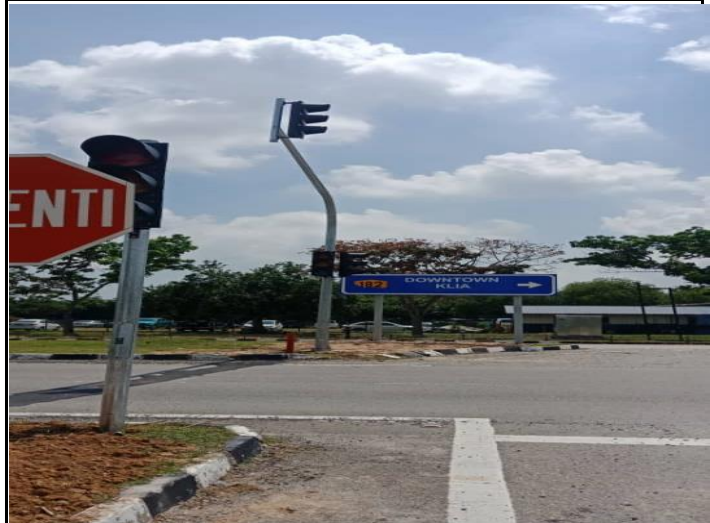
complete to install overhead pole and normal pole
