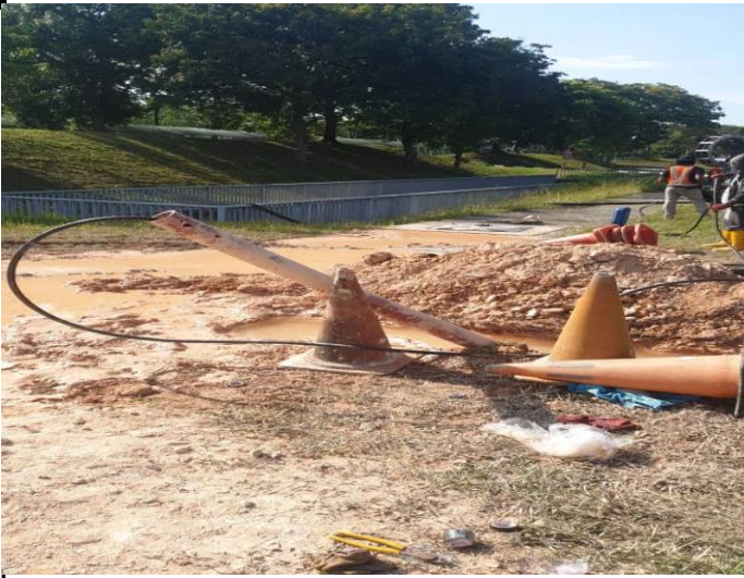
completed to lay the pipe and power cable
