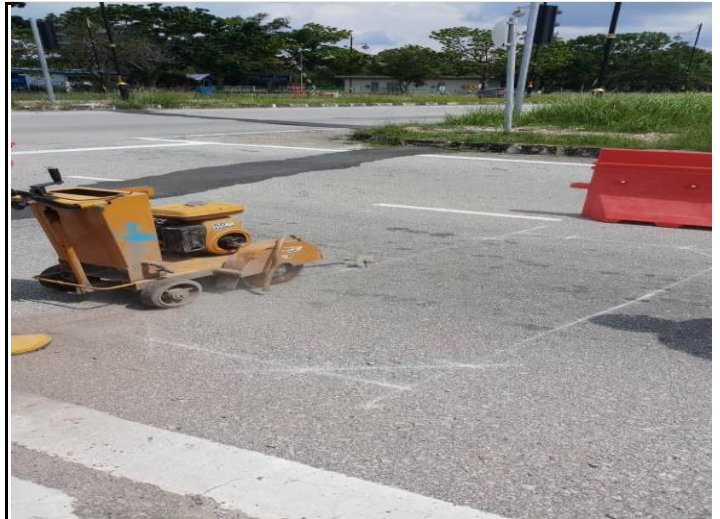
prepare cut the road to lay the loop cable
