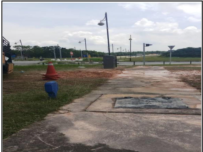
site clearing after lay pipe
